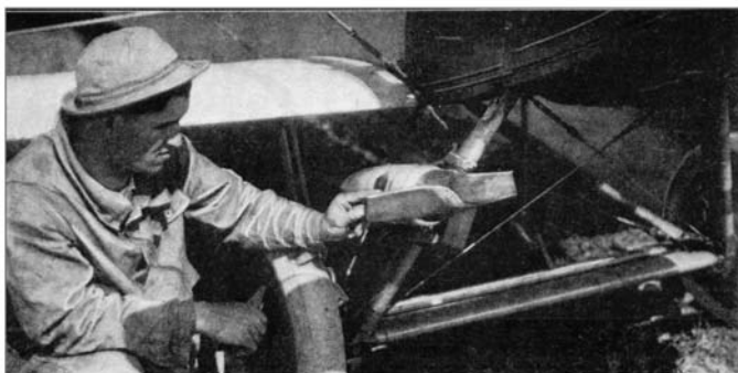
Inspecting the GN-1 Generator Used For the Wireless Telephone System.
