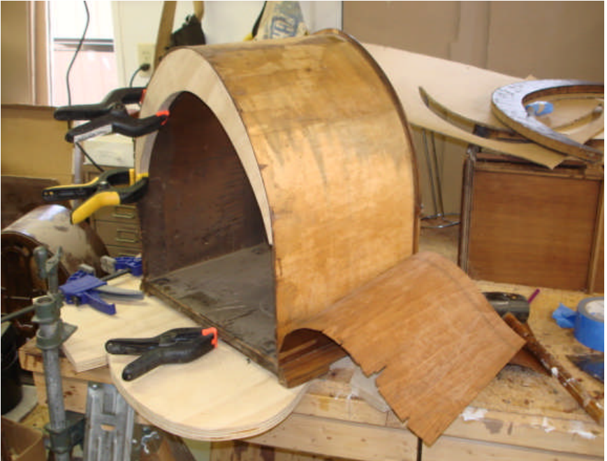
In the above photo the replacement arch is being fastened to the top of the cabinet.
