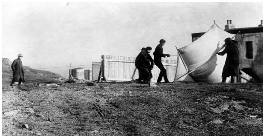
Marconi watching associates raising the kite (a "Levitor" by B.F.S. Baden-Powell) used to lift the antenna at St. John's, Newfoundland, December 1901.
