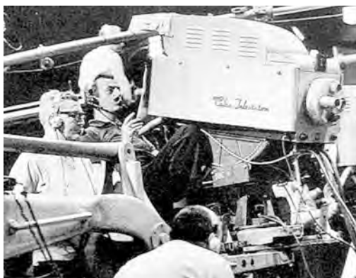
TK-41 in use during a 1960s Hallmark Hall of Fame production at NBC studios in New York. Note the kludged viewfinder hood. It is quite common to see the stock RCA-supplied viewfinder snout either removed or replaced by a different hood more to the liking of the camera operator.
