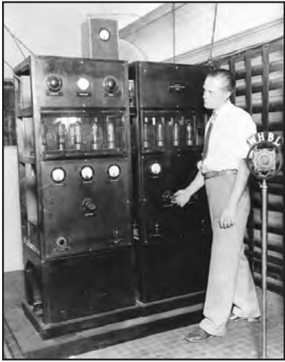
July 1, 1927: WHBL, one of Charles L. Carrell's portable stations, was installed in a special railroad car of the Chicago, Milwaukee and St. Paul Railroad's express train, the Pioneer Limited. Engineer K. W. Pyle adjusts the transmitter.
