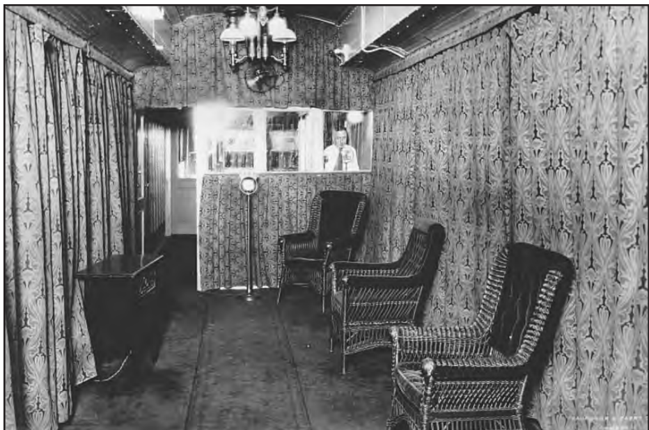
This view shows the studio half of the railroad car of radio station WHBL. A complete radio program was broadcast from here while the train was en route from Chicago and Minneapolis on July 1, 1927.
